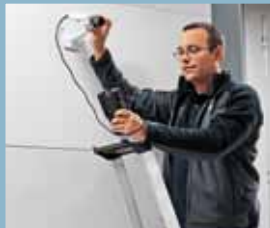
Mount the cameras and install cabling
